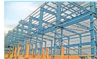
Steel Pipe Factory (Nippon Steel - Japan)
