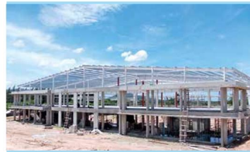
Ticon Logistic Warehouse (Thailand)
