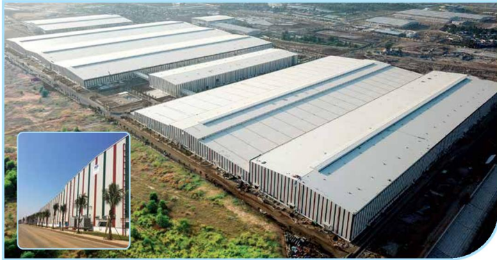
VinFast Automobile Manufacturing Complex (Haiphong - Vietnam) - 14,000 MT
