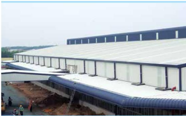
Beesco Vina Binh Phuoc - Water Distribution Tray
