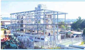
Six - Floor NMMC Hospital (Philippines)
