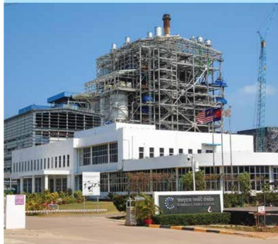
Narawat Power Plant (Cambodia)
