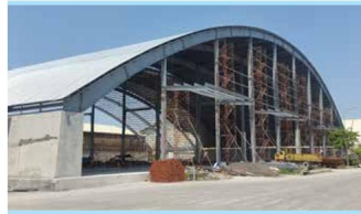
NPK Warehouse, Wilmar Project (Indonesia)
