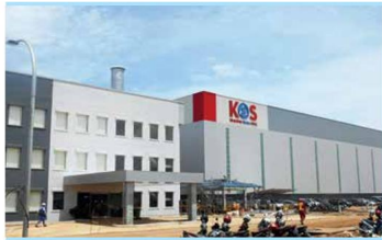
Krakatau Osaka Steel Mill (Indonesia)
