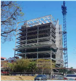
14-floor Workspace Building (Philippines)
