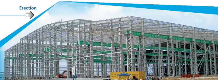
Heavy Steel Structure Factory (Doosan - Korea) - 11,300 MT
