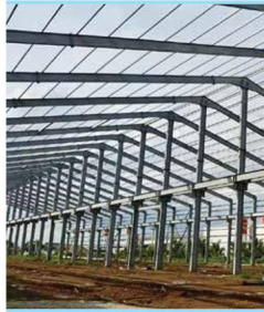
SJC Concrete Warehouse (Thailand)
