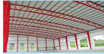
Jade Land Warehouse (Myanmar)
