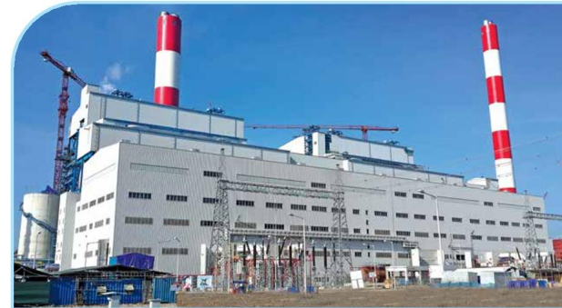
Siding Works Project of Mong Duong II Power Plant (Doosan) - 50,000m 2 Using Hyper180™ Panel (AZ180 Coating + PVDF Paint)
