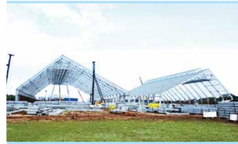
Flat Storage, Krakatau Bandar Samudera, Cilegio (Indonesia)
