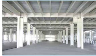
Mezz: Column, Beam, Joist, Deck
