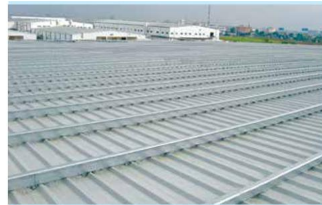
Composite Roof with Sub Purlin
