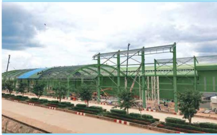
FCB Warehouse Phase 2 (Thailand)
