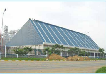
102% Roof Slope, SoyBean Meal Factory (Baria Serece)
