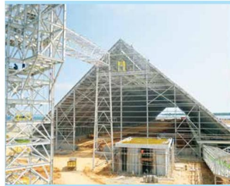
85% Slope for Fertilizer Storage (PT Pupuk Kaltim - Indonesia) - 1,650MT
