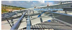
Galvanized Flange Bracing
